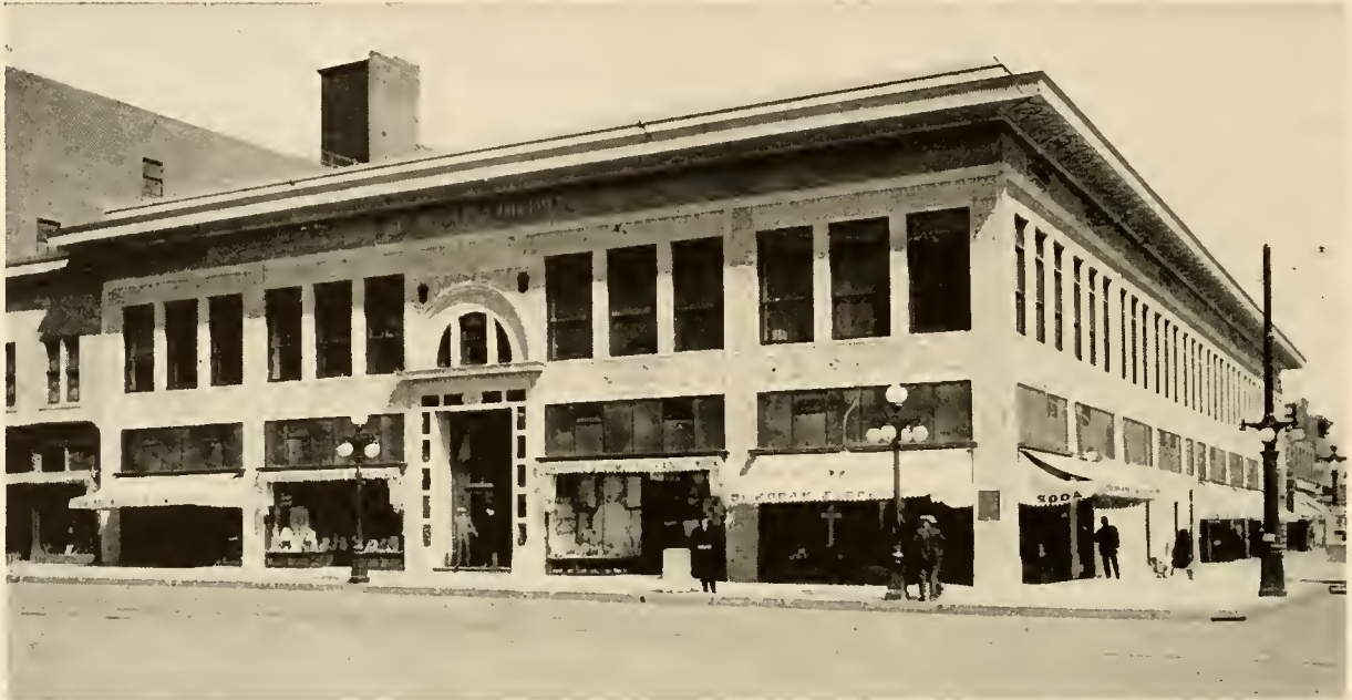
STRATTON STORE BUILDING, COLORADO SPRINGS, COLORADO
